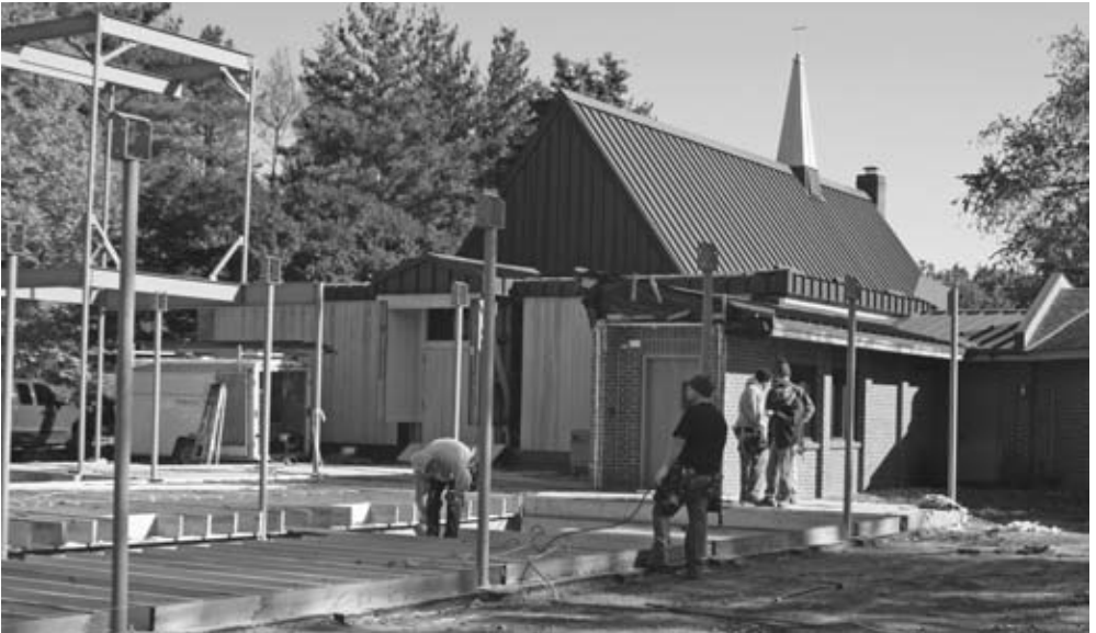
Construction continues on our new bell tower and church entrance.
